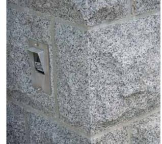
Local, Cape Ann granite of homogenous color was the specified material for this pier construction. To satisfy this challenging request, our boom truck ultimately served as a derrick to extract two freshly quarried blocks which were used to fabricate the pier caps. Several weeks of profiling and intricate hand-tooling resulted in a new-stone construction that not only serves the design, but respects the local culture and topography.
