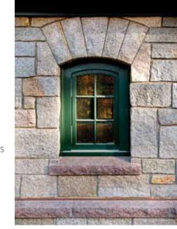
One-hundred arch stones serve as the defining feature of this carriage house. Each was excavated painstakingly from material sometimes as much as three times their finished size. In total, over four hundred tons of raw material was sourced and salvaged to complete this concept.
